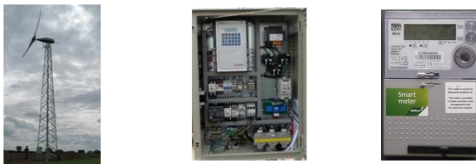
Figure 11: 11kW wind turbine with associated control panel and smart meter
